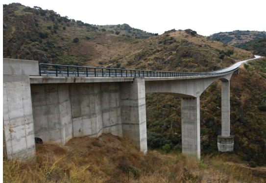
a) General view of the bridge
