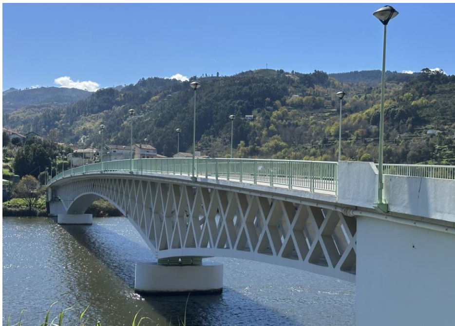
Figure 1. General upstream view of the Mosteirô Bridge, from the north bank.
