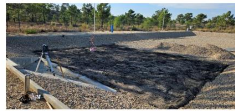
Figure 2.5 Aspects of the placement of the two reactive organic layers in Basins 1 and 2, at Comporta WWTP_SAT-MAR
