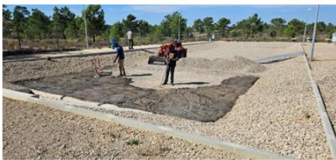
Figure 2.5 Aspects of the placement of the two reactive organic layers in Basins 1 and 2, at Comporta WWTP_SAT-MAR
