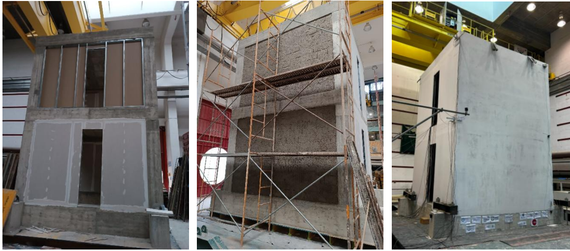
Figure 3: From left to right: construction of plasterboard infills, construction of brick infill walls; prototype completed in FB configuration.
