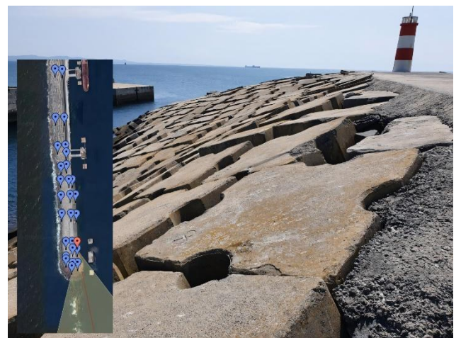
Figure 7. 2020 visual observation at Point 28F of Sines west breakwater (inner armour layer)
