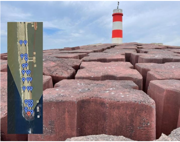
Figure 8. 2022 visual observation at Point 37T (T – Back direction) of Sines west breakwater (head, section I)
