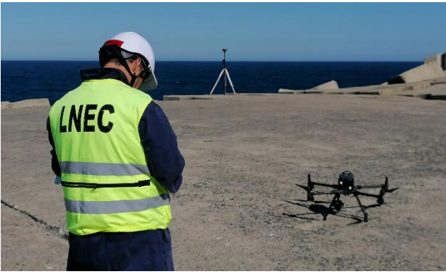
Figure 14. Drone operator preparing the flight on Sines west breakwater. Shown on top of this image is the RTK GNSS antenna base
