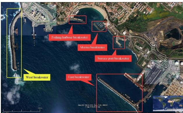
Figure 2. Rubble-mound breakwaters in the port of Sines
