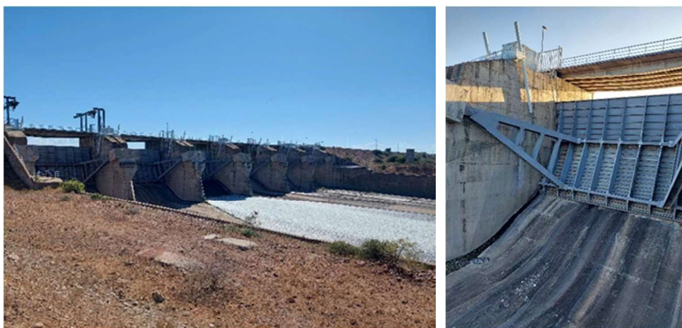
Figure 11 – Downstream view of the spillway crest and detail of a spillway gate
