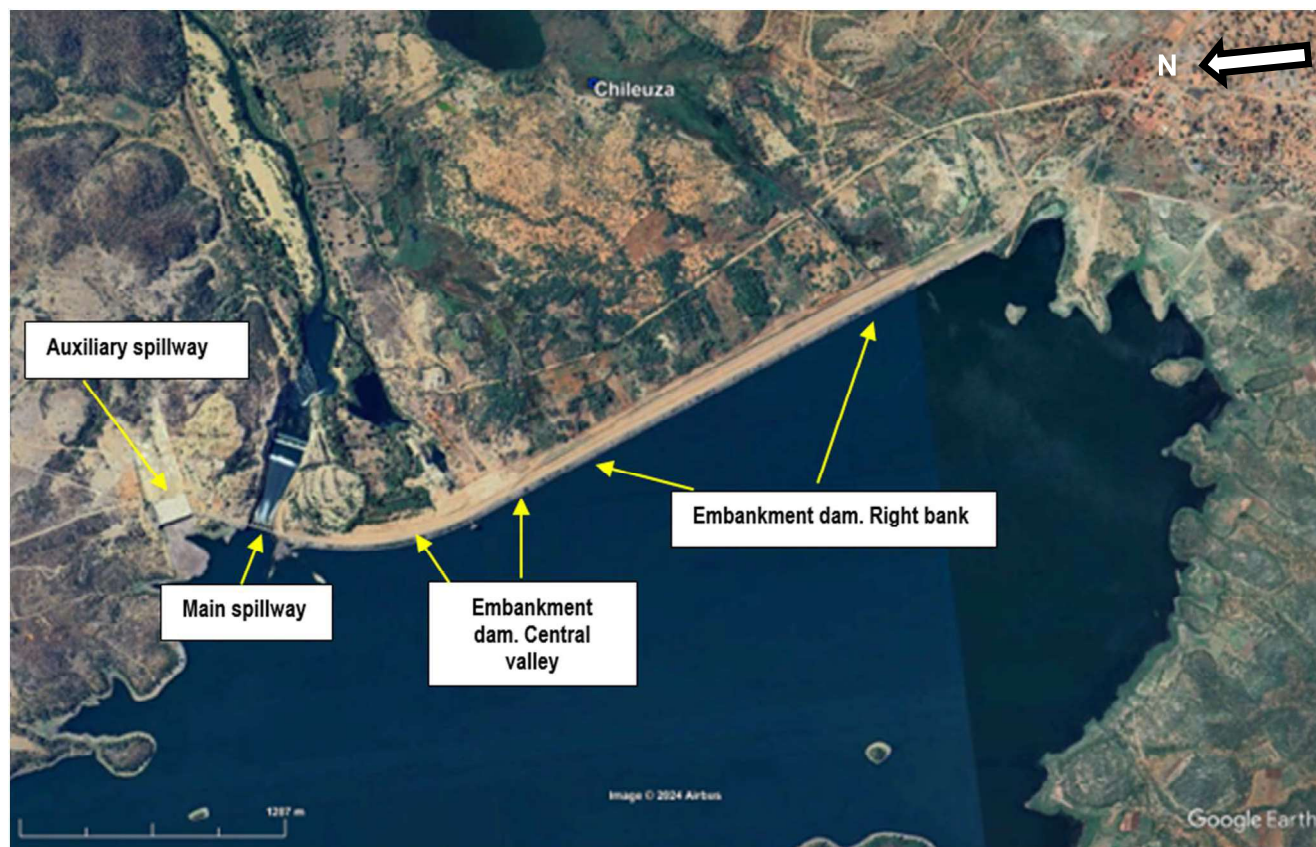
Figure 1 – Massingir dam general view (google earth).
