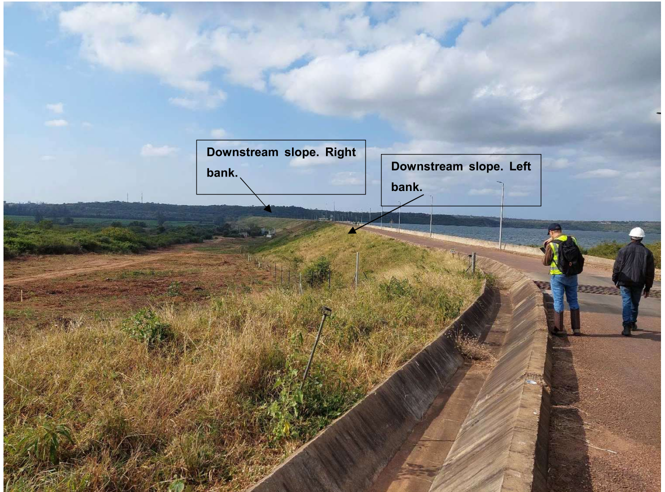
Figure 6 – Downstream slope. General view (view towards the right bank).
