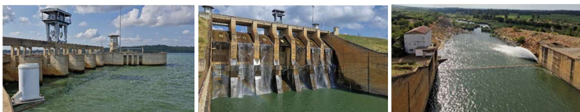
Figure 1 – Appurtenant structures. Upstream and downstream views
