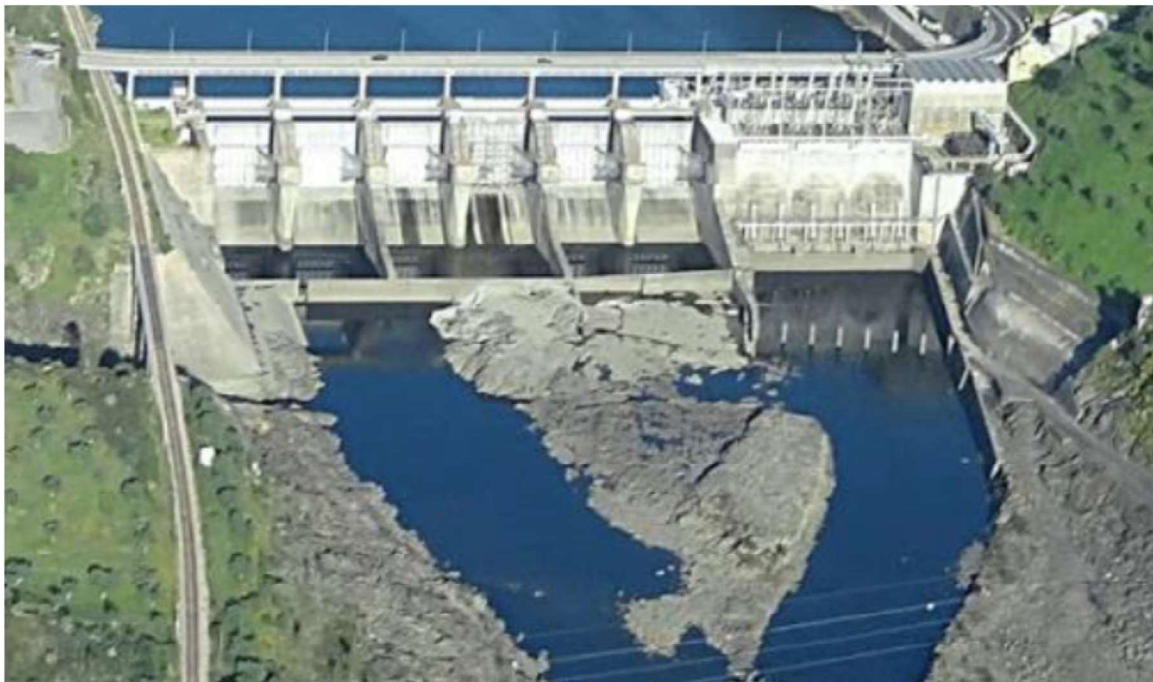
Fig. 2 – Overview of the Fratel Hydroelectric Scheme from downstream [8]
