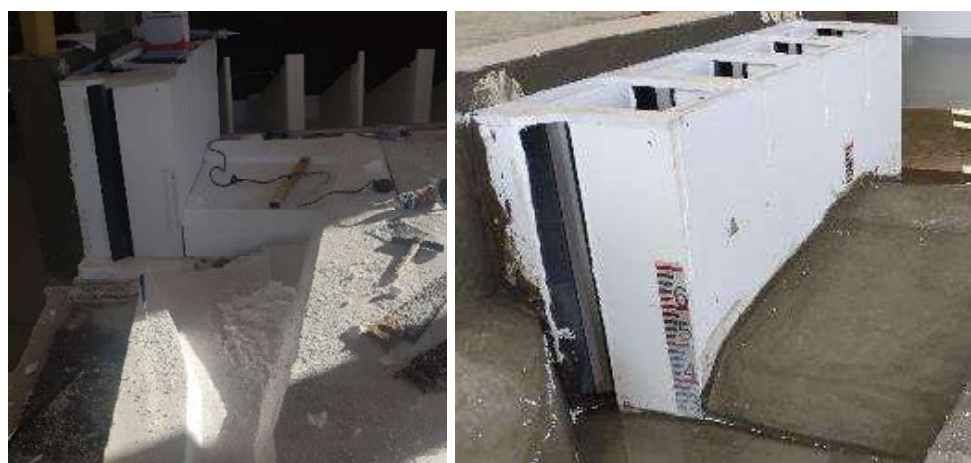
Fig. 10 – Physical model construction: fishway and bypass channel
