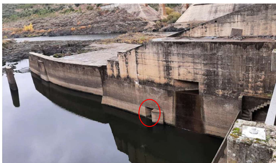
Fig. 4 – Fish lock entrance: view from the tailrace structure of the generating units [8]
