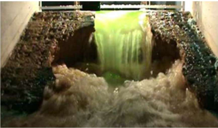
dam & dike erosion
