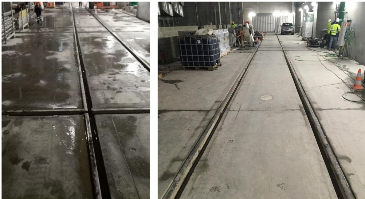
Fig. 9 – Floor slab of the transformers cavern before (left) and after (right) waterproofing works and collecting water
