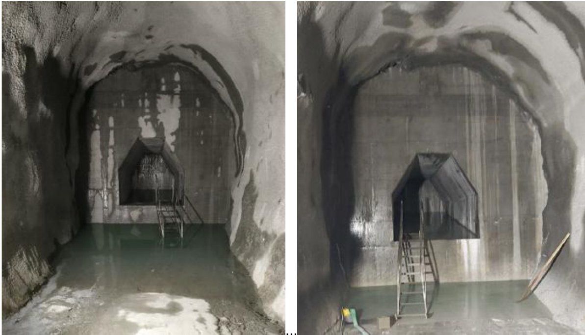
Fig. 10 – Lower plug before (left) and after (right) pumping the inflow water to the access tunnel
